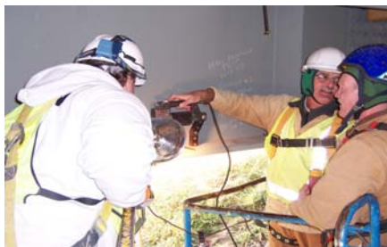
Mike Ohanian and Frank Martin Conducting a Weld Inspection Dayton Expressway Bridge
