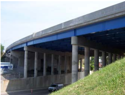
Dayton Expressway Bridge After Construction
